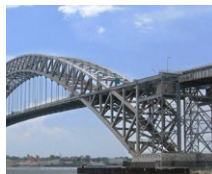
Bayonne Bridge (US)
