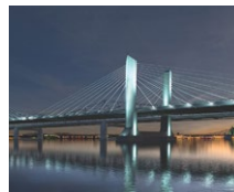
Ohio River Bridge (US)
