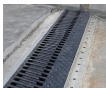
Sliding Finger Joints
