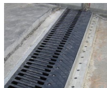
Sliding Finger Joints
