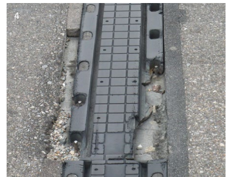
1 TENSACRETE expansion joint RE type 2 TENSACRETE expansion joint RE-LS type 3 Damaged bituminous expansion joint 4 Damaged mat expansion joint
