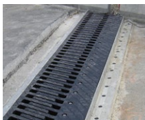
Sliding Finger Joints
