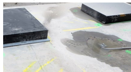
VIBRAX®BLOCK B vertical bearing ready for the load distribution plate
