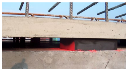
VIBRAX®BLOCK B bearing under load distribution plate
