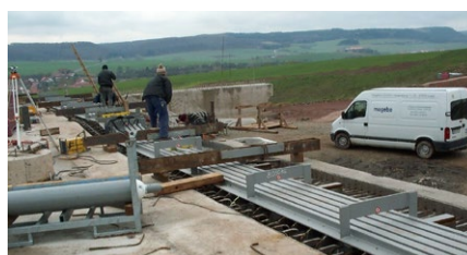
Installation of a TENSA®MODULAR expansion joint on the bridge in 2002
