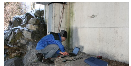
Installation of the ROBO®CONTROL automated monitoring system
