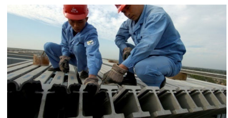
TENSA®MODULAR expansion joint type LR24 ready for installation
