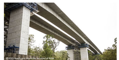
The Hunter Expressway viaducts over Sugarloaf Range with its steep gullies.
