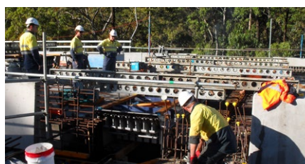
A mageba TENSA®MODULAR expansion joint during installation on the first viaduct
