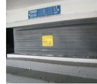
Elastomeric bearing
