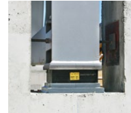
Reinforced elastomeric bearing
