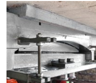
Cylinder bearing
