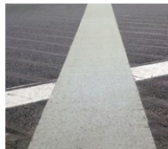
Flexible plug joint
