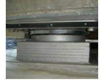
Spherical bearing
