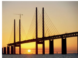
Öresund Bridge, Denmark
