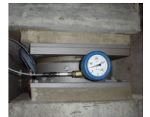
Lifting and measuring bearing
