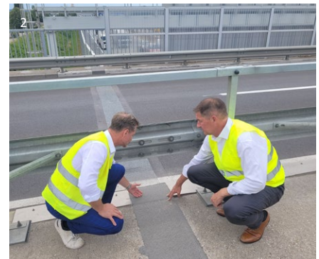
Sliding finger joint
