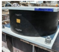
Lead Rubber Bearing (LRB)
