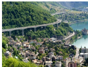
Viaduct de Chillon, Switzerland
