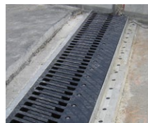
Sliding Finger Joints
