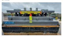
An installed spherical bearing that supports the roof structure of the sport complex
